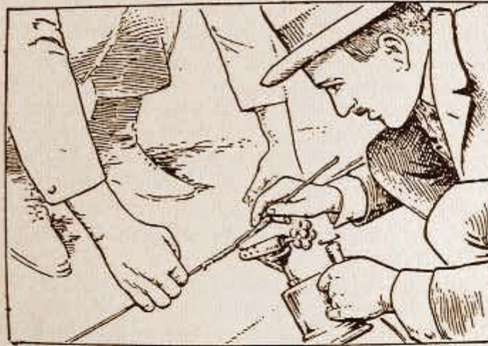
Fig. 117.—Soldering ground wires with torch.
